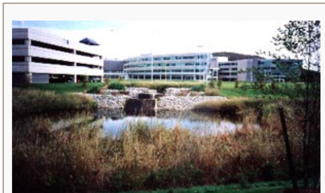
A stormwater detention pond is constructed and wetland plants are established using Agresoil Compost™.
